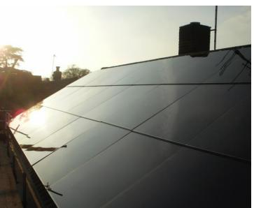
Polysolar's PS-A glass panels incorporate amorphous silicon technology to achieve
